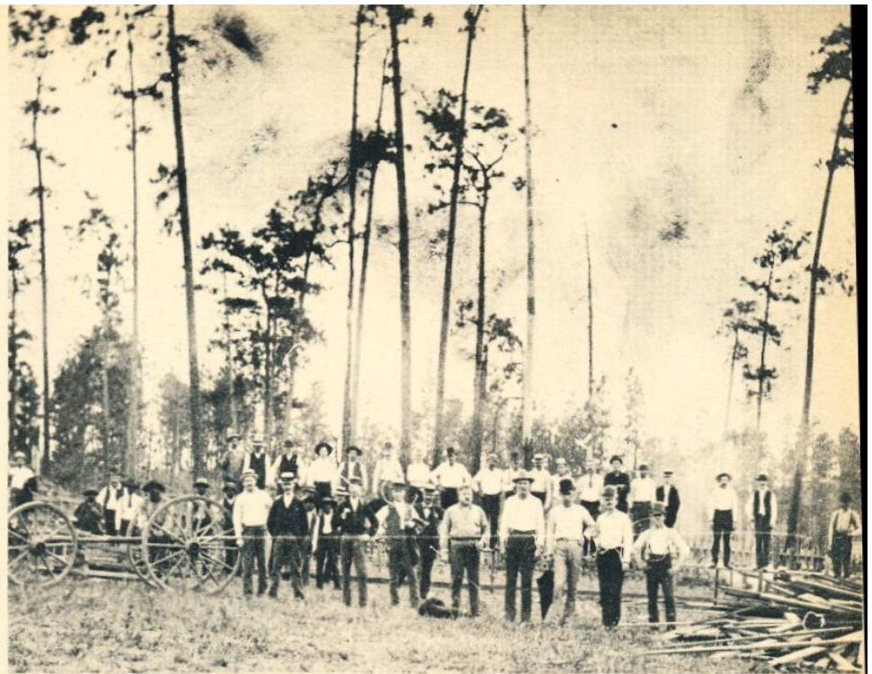
Pye's camera captures construction crew which built enclosure where the fight took place. Picture was taken on the morning before the fight.
